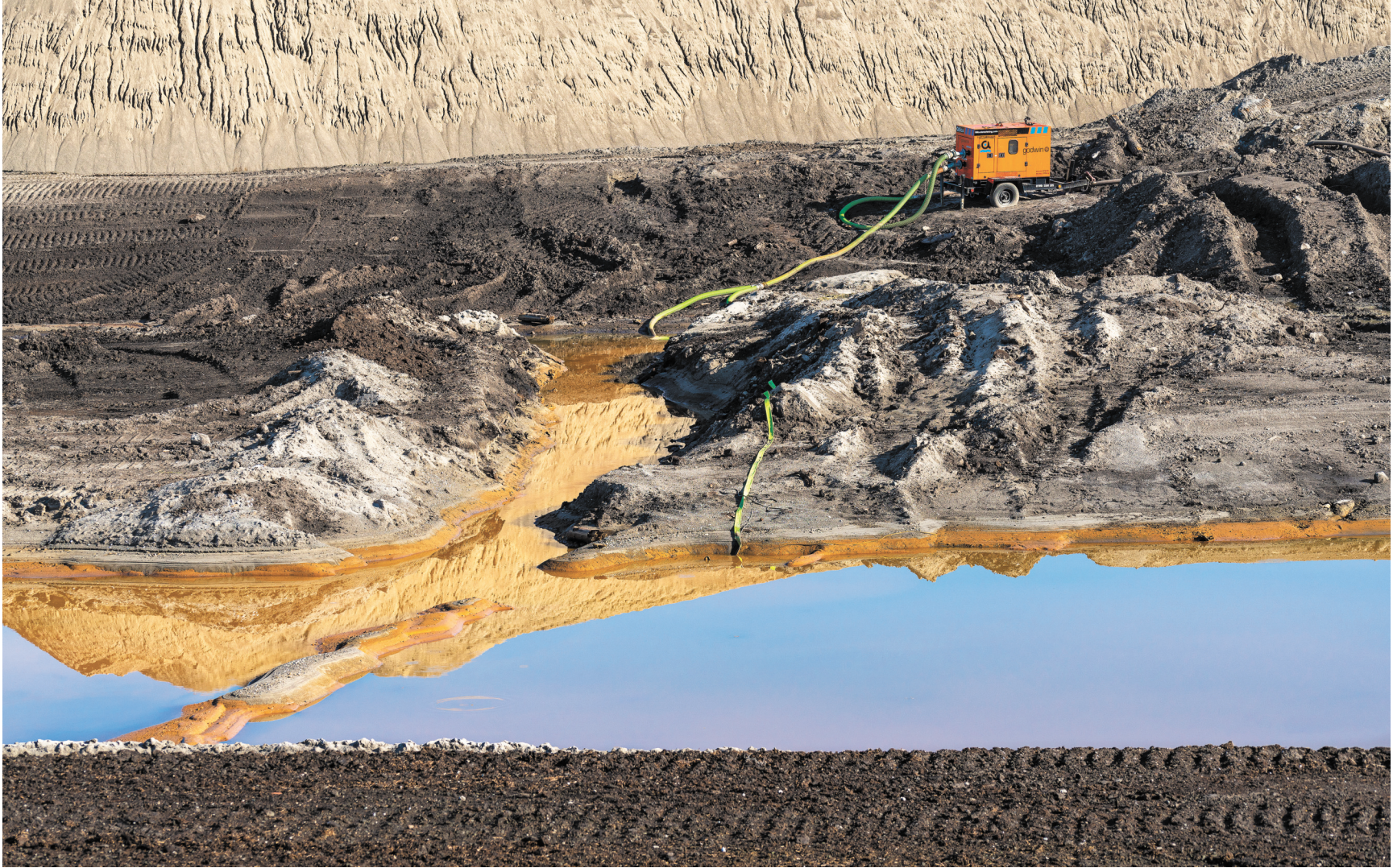
Early in our six-year commission, we witnessed the constant movement of vast mounds of carefully categorized soil around the site as the new river valley was being excavated. Here water is being pumped out of the excavation and this scene itself no longer exists but is likely now part of the new river bed.
